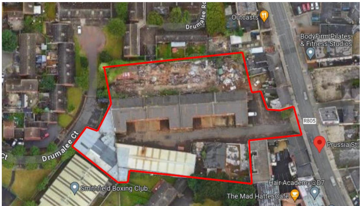
Figure 1 Development Site at Prussia Street, Dublin 7
